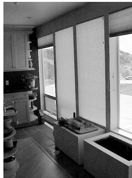
Windows from the inside, covered with special insulating blinds.
