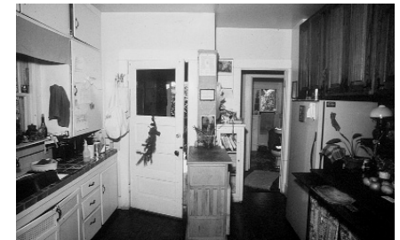
South view of kitchen before renovation
