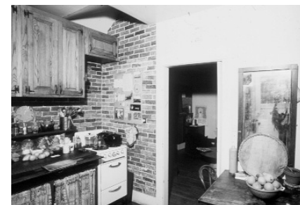
Northwest view of kitchen before renovation
