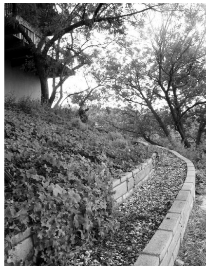
Rainwater dispersal system
